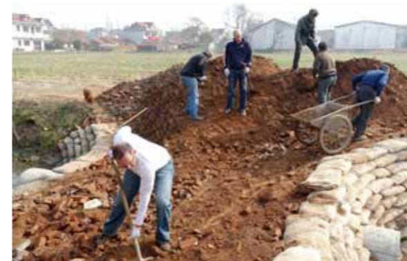
CONSTRUCTING THE BRIDGE AT GEP4
