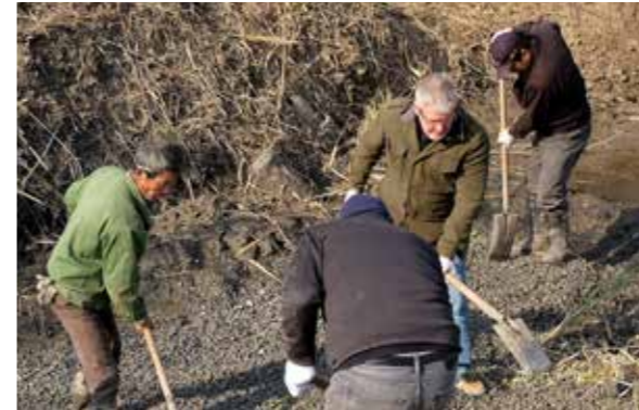
CONSTRUCTING THE BRIDGE AT GEP4
